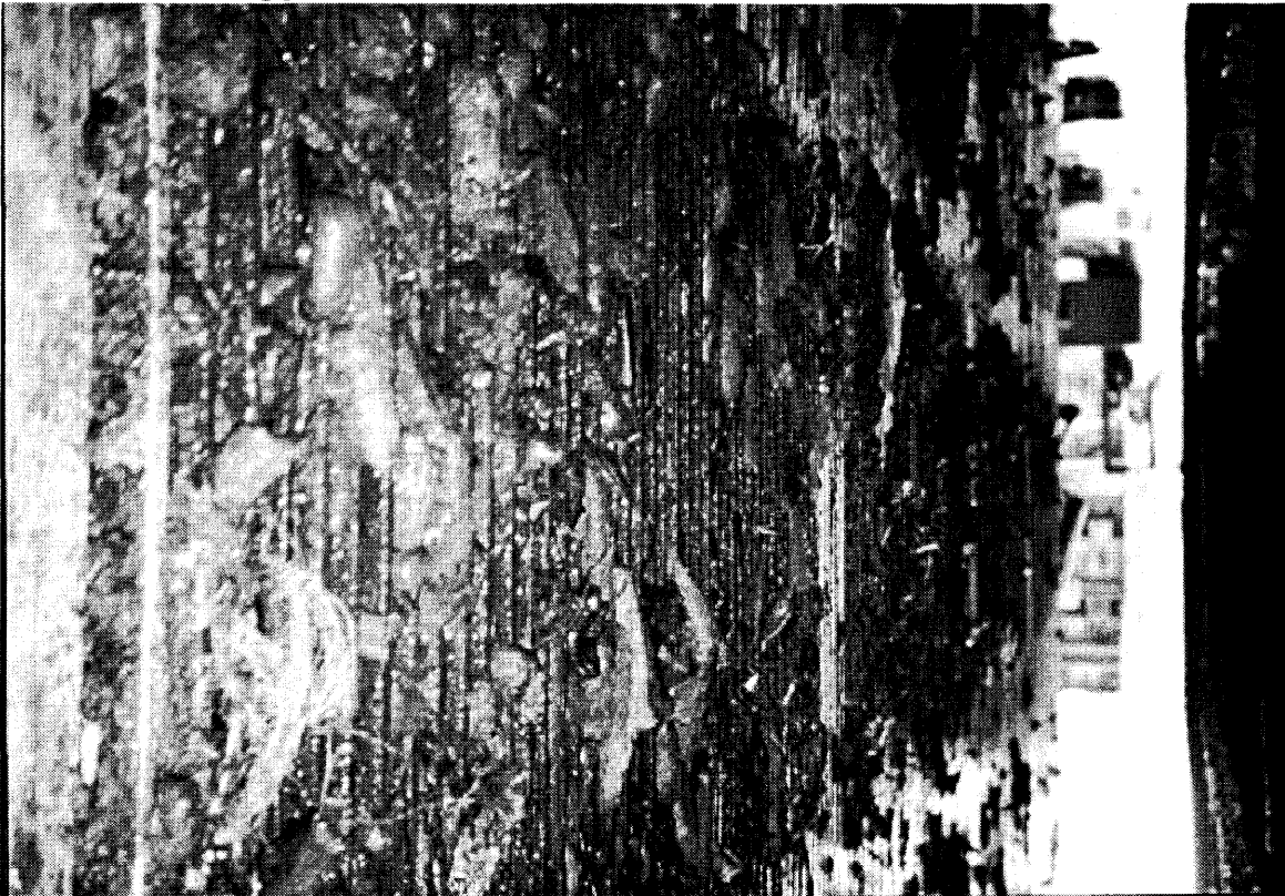
Photo 4. Debris Clogged Fish Unit Trash Rack
