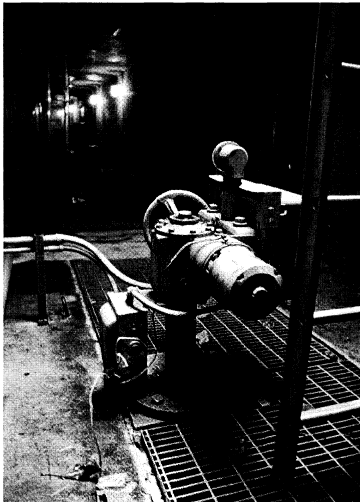
H5 Diffuser B Gate Actuator
