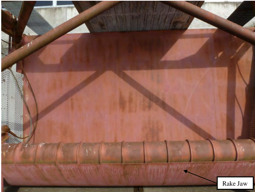
Figure 5-2: Front of Existing Rake
