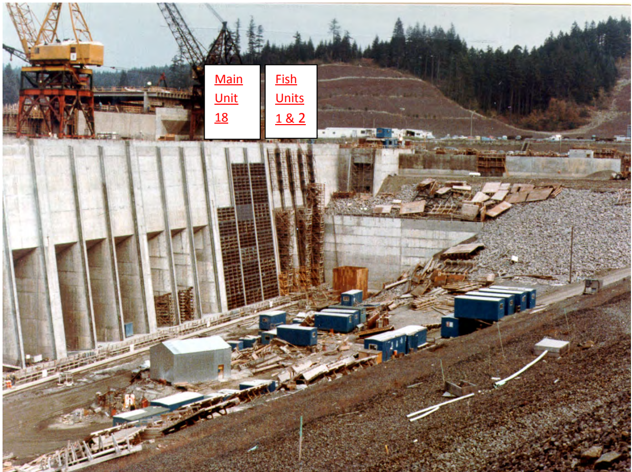
Figure 2-5: Bonneville Dam Fish Units (Adjacent to Wall) During Construction
