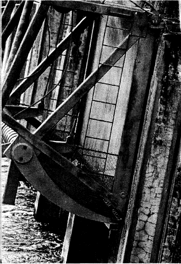
H1 Existing Rake
